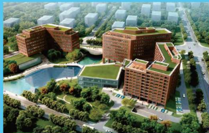
1、青岛中德生态园被动房技术体验中心 Qingdao Sino-German ecological park passive house technology experience center
